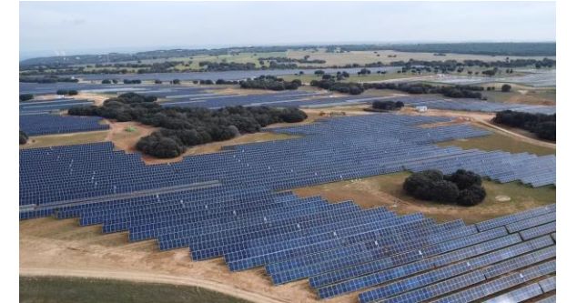
1st flagship 626MW Trillo PV plant 476MW in operation/150MW under construction
