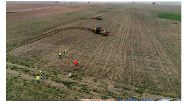
2nd flagship 700MW Garoña PV plant Start of civil works
